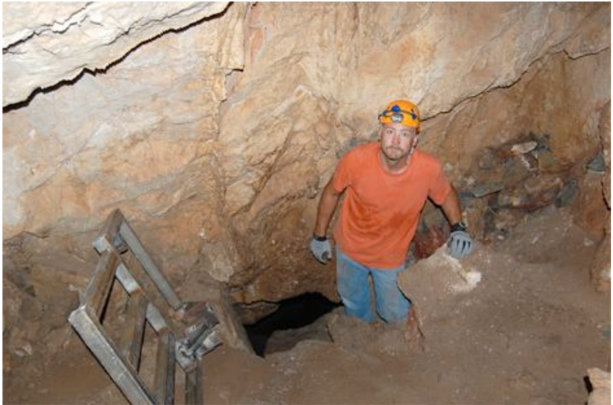
Gate Inside of Cave and Ready for Placement
